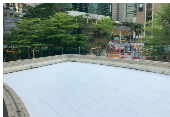
Rooftops coated with “electricity-free cooling technology” paint, the Gold Award-winning project, can significantly reflect heat and reduce the energy consumption of the buildings for cooling.
